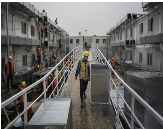
Wuhan New Hospital construction
